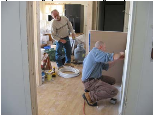
Gary (Grampie) and Sean at work on the renovations
