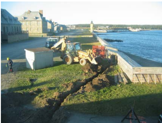
Pictured above is the work in progress
