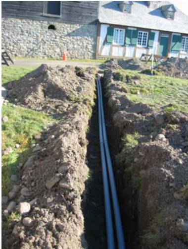
Line completely installed.
