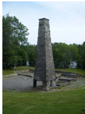
Remains of the first iron works in Canada, 1730 Les Forges du Saint-Maurice NHS
