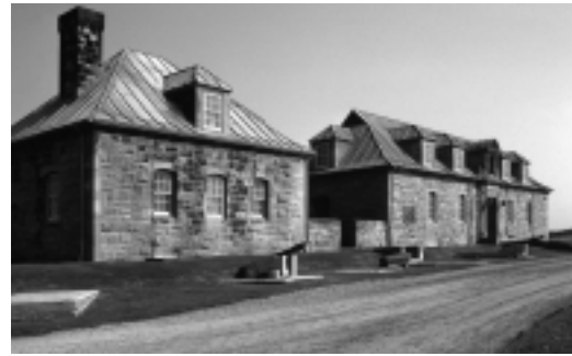
IMAGE 9. Museum and caretaker's house
