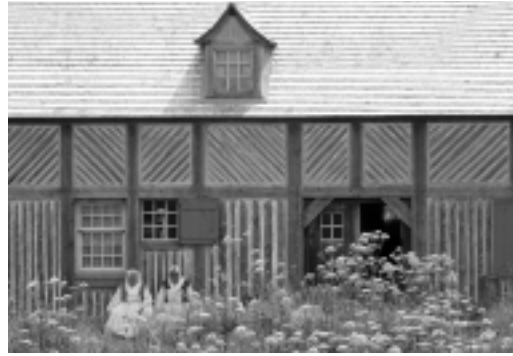
IMAGE 55. Timber frame building with "piquet" in-fill
