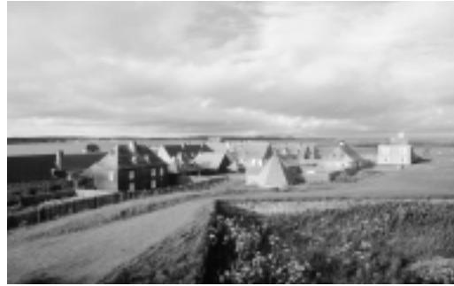
IMAGE 13. View of reconstructed townsite
