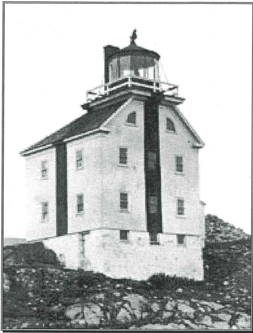
The Louisbourg Lighthouse 1842-1923, south side. The lighthouse was wood frame, shingled and painted white with a black vertical line on three sides. It was 35 feet high to the vane on a 29 foot square, stone foundation. Photo taken after 1889.
